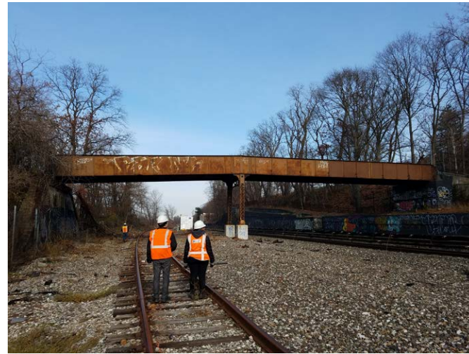
Photo A09: College Point Bridge near West 261st Street
