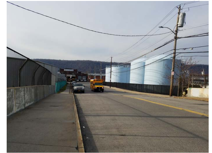
Photo A11: Ludlow Street Bridge over Metro-North tracks, looking west
