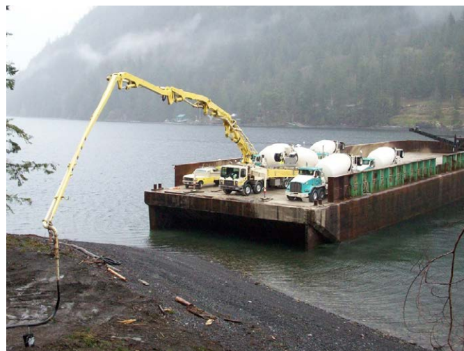
Photo A18: Example of concrete installation by barge
