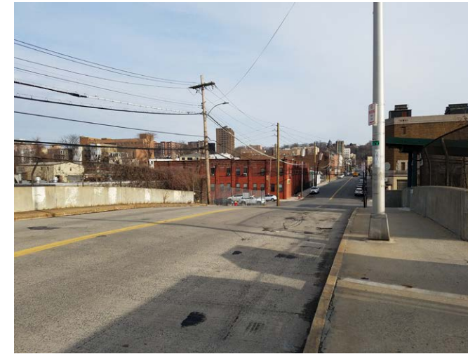
Photo A10: Ludlow Street Bridge over Metro-North tracks, looking east
