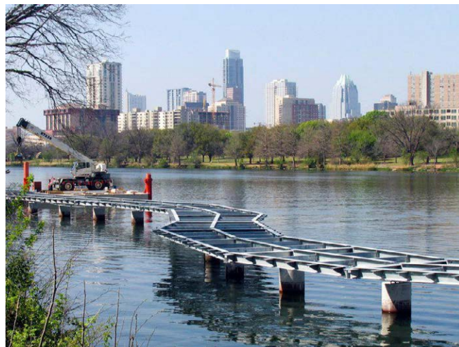
Photo A15: Example of construction of elevated walkway from barge
