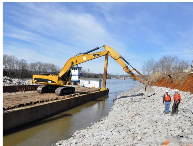
Photo A16: Example of rip-rap installation from a barge
