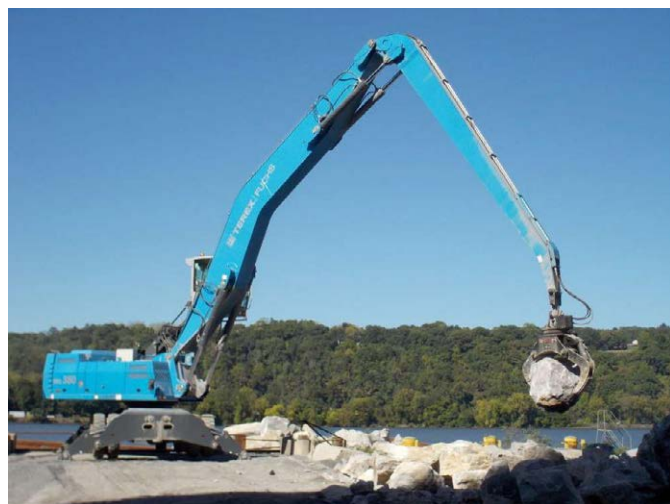
Photo A17: Example of placement of large rip-rap
